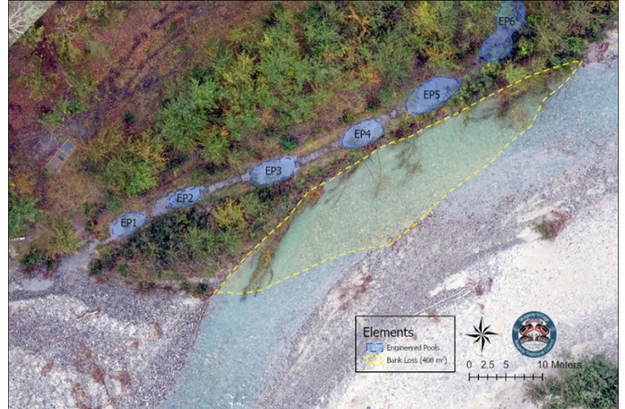
Aerial imagery of the Skagway River engineered fish pools near Seven Pastures
